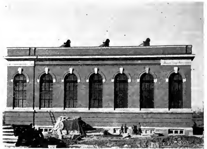
View of the Substation at Mount Royal Model City.
